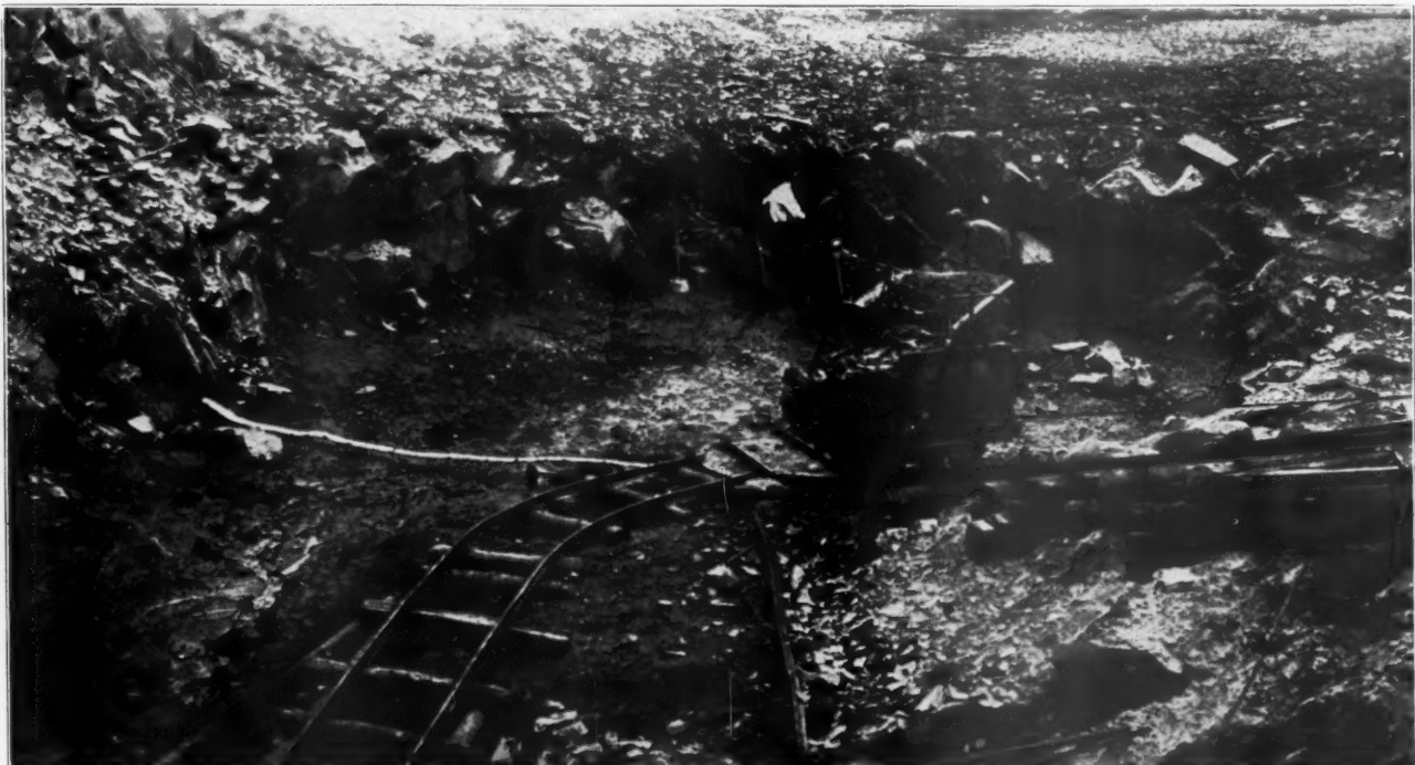
View of Quarry Showing White Quartzite Being Loaded Into Dump Cars
